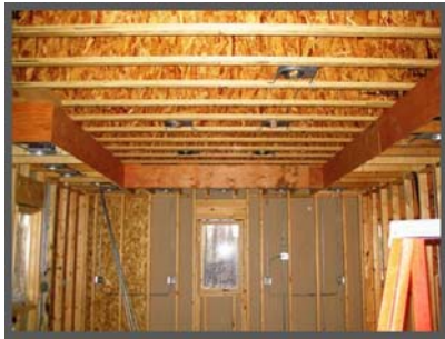
Residential construction: Mostly dry materials invisible to RF signals
