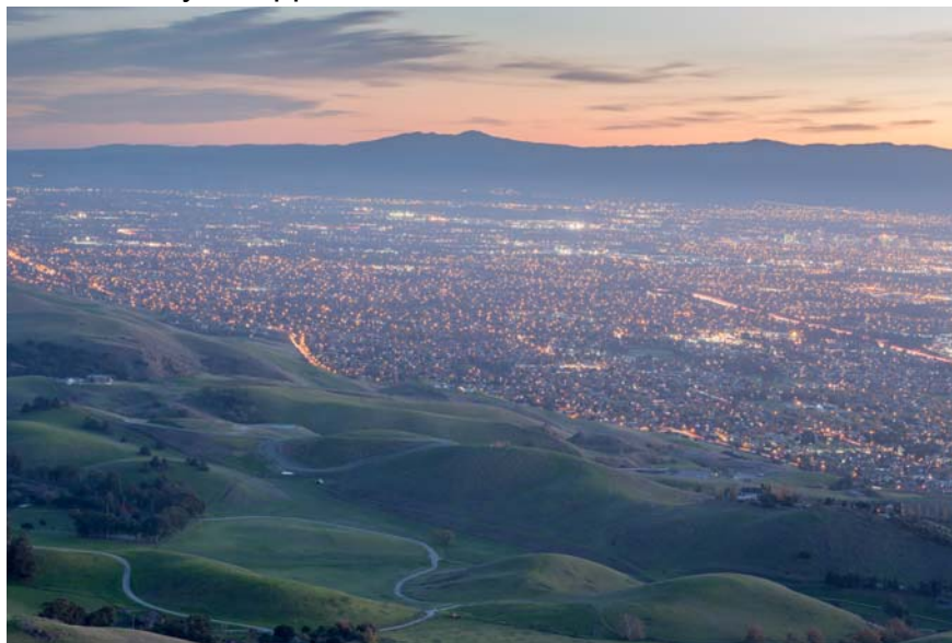
Figure 1 A 2013 attack targeted a substation which provides electricity to Silicon Valley
